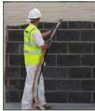
Monocouche render must be mixed with consistent volume of water throughout the application and across all areas, this requirement and increased output and efficiency is the reason that we state that application by render machine is best practice however with experience it can be mixed using a cement or paddle mixer and applied with conventional hand (hawk and trowel) methods.
