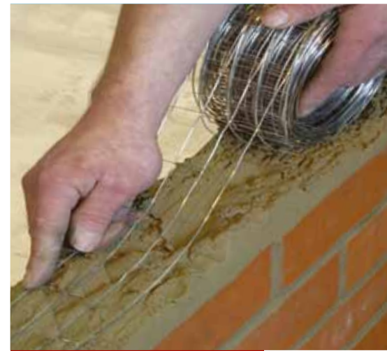
Standard masonry joints
